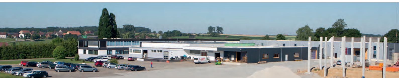
2018: new Mechanical Plant with 1.600 m 2
