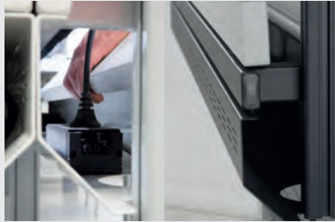
spacious cable tray 200 x 170mm for cable bundles or battery chargers, etc.
