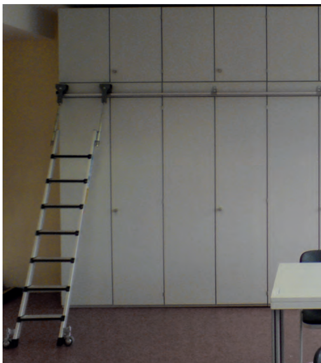
rail system with extensional ladder and casters
